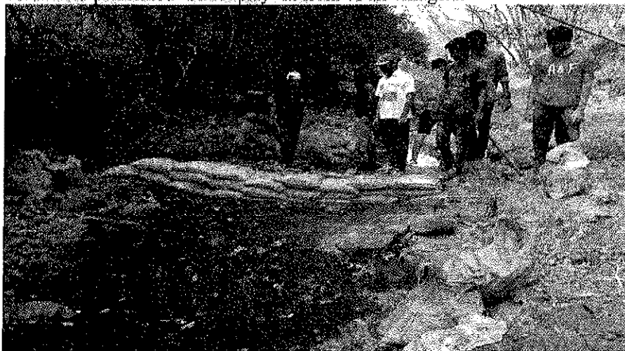
VanraiBandhara construction
