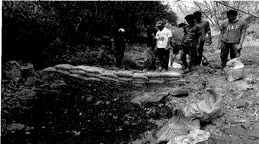
VanraiBandhara construction
