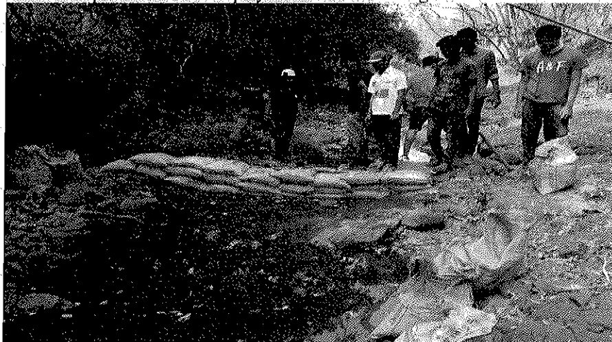
VanraiBandhara construction
